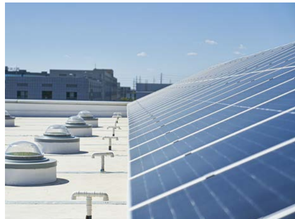
The Shenyang plant features light chimneys and on-site solar panels.
