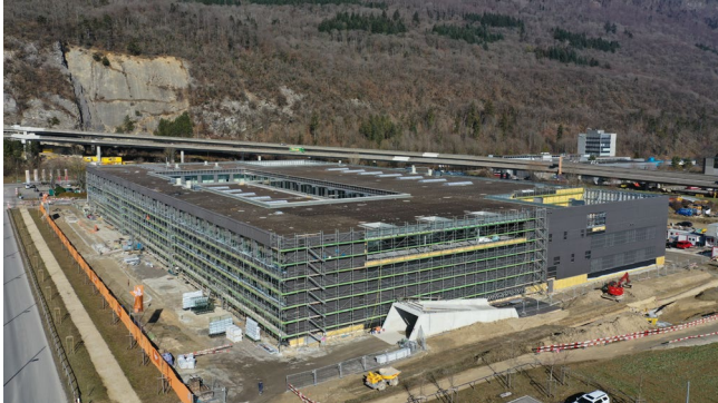
Innovation and production center, Biel, Switzerland
